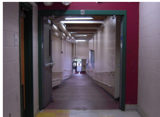
Ramp down to lower gym
