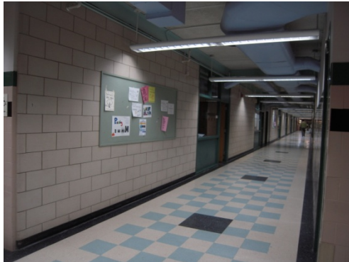
Corridor: glazed block, exposed struct. & MEP
