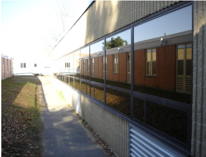
Figure 17. Typical window wall at Building L from 1970s construction.
