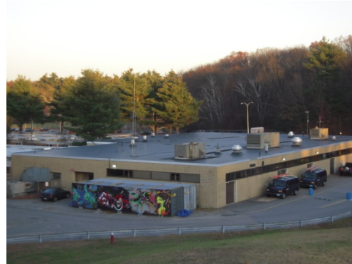
West and south side view of building I
