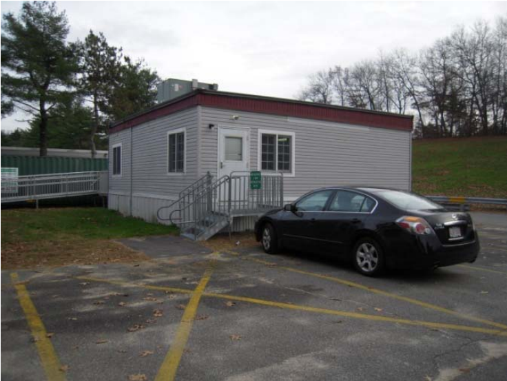
STAND ALONE CLASSROOM TRAILER OUTSIDE OF UPPER GYMNASIUM
