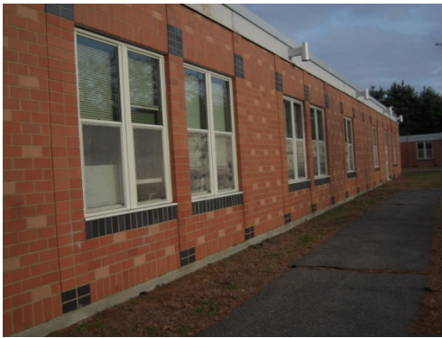
Brick veneer with punched window openings
