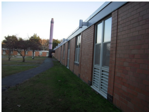
Brick veneer with punched window/louvers
