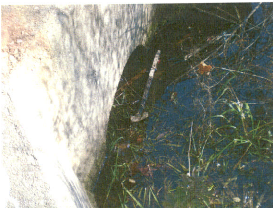
Culvert under Thoreau Street to wetland
