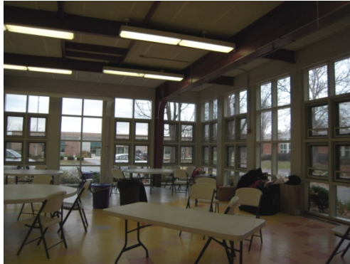
New VCT cafeteria floor and exposed structure
