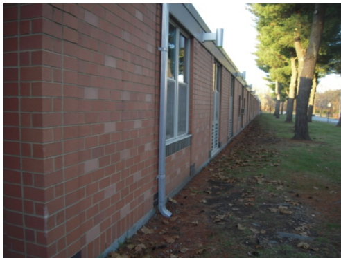
Brick veneer with punched window/louvers
