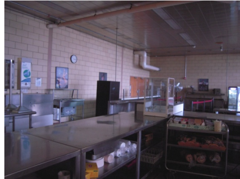
Glazed block walls in kitchen and S.S. ceiling
