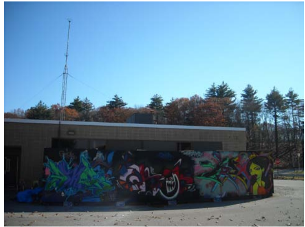
Gas Fired Rooftop Unit - Building I
