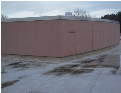
Metal panels at auditorium and PVC roof
