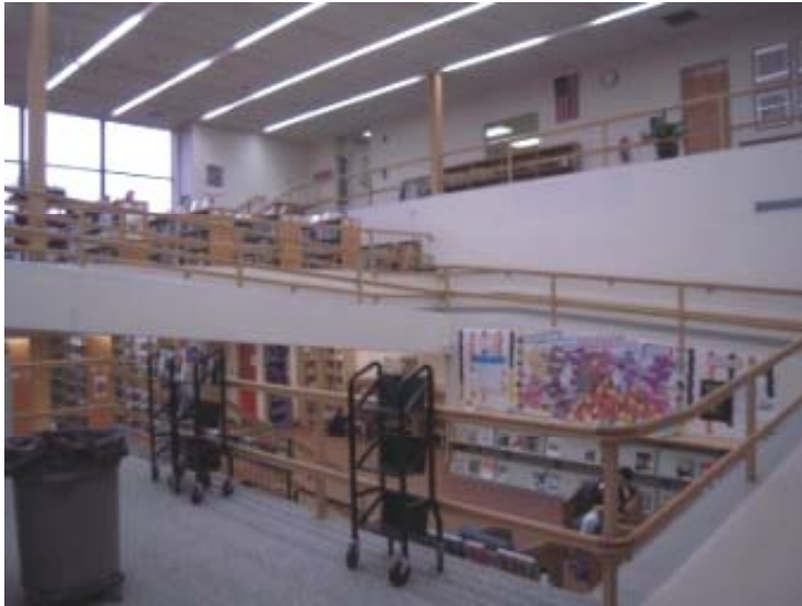
NONCOMPLIANT RAMP IN LIBRARY
