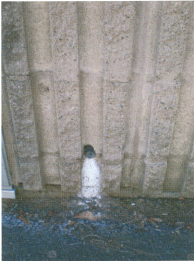
Weep holes at face of L-Building
