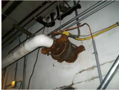
Main water service
