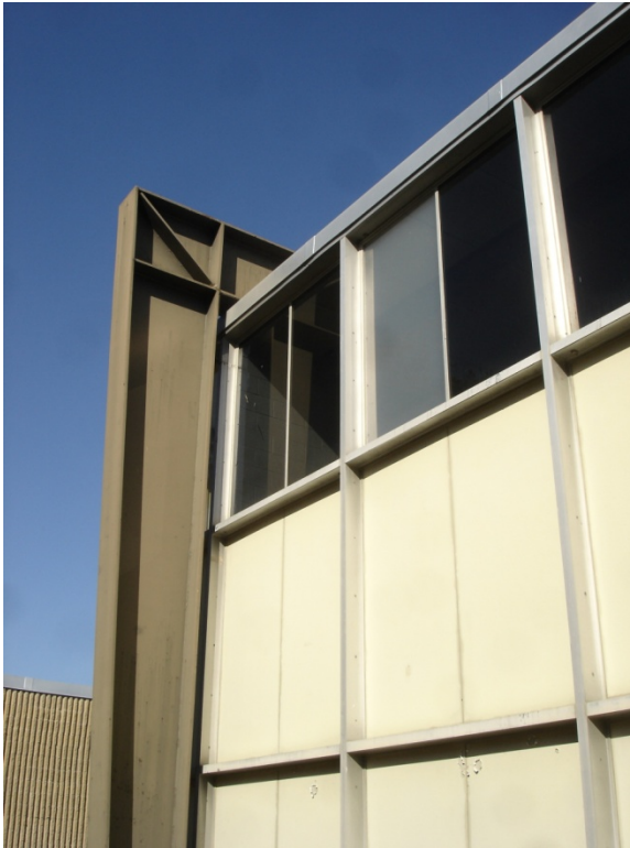
Figure 23. Exterior curtain wall at upper gymnasium.
