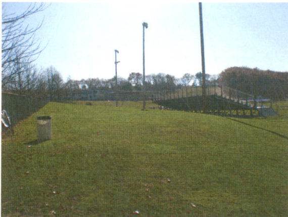
Sewer location behind bleachers
