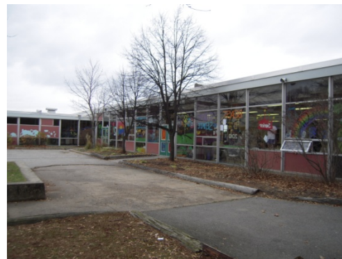
Original curtain wall system on south side of cafe.
