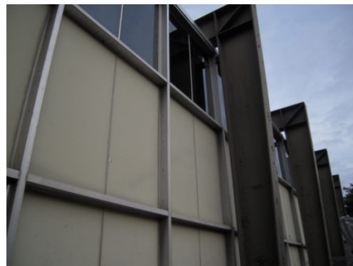
Exposed performance gym structure & curtain wall
