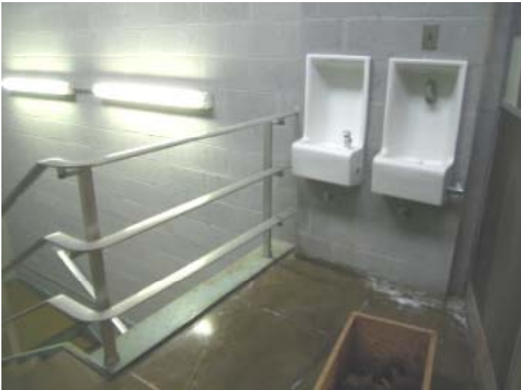
NONCOMPLIANT GUARDRAILS AND RAILINGS IN STAIRWELLS / DRINKING FOUNTAINS DO MEET CODE REQUIREMENTS
