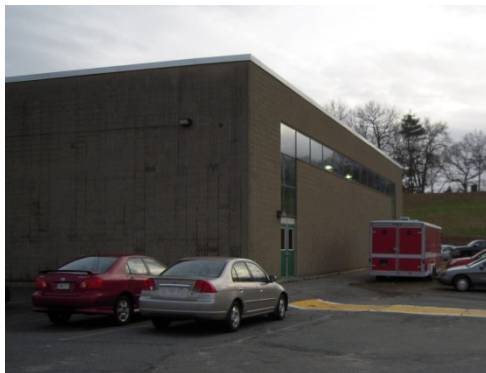
North and west wall at lower gym
