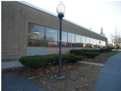
Spilt faced ribbed block and aluminum storefront
