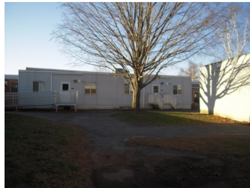
Classroom trailer outside of building I
