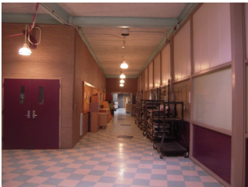
Exposed ceilings, paneled walls, VCT flooring
