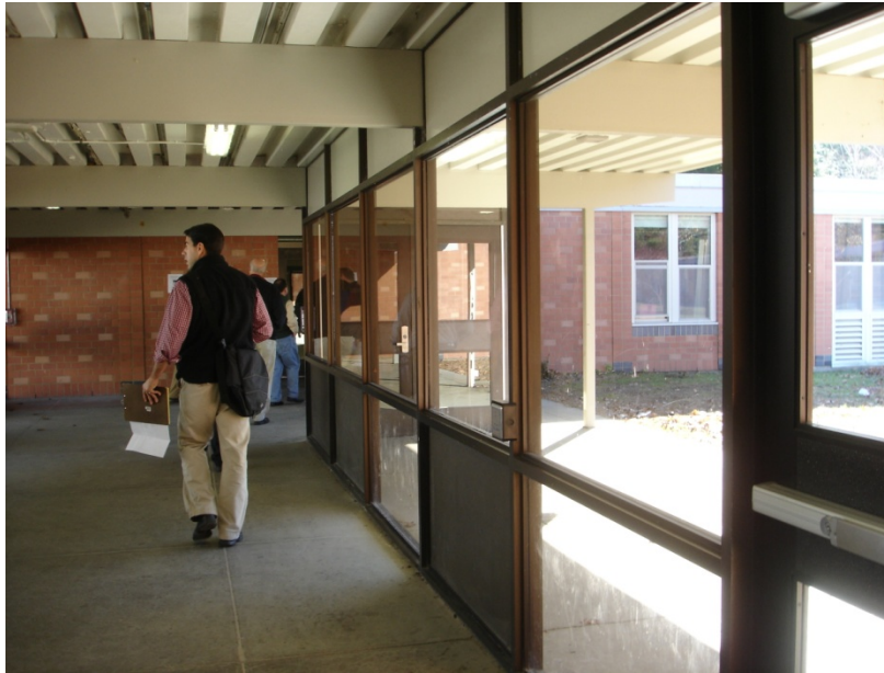
Figure 13. Typical single pane curtain wall at breezeway between buildings A and S. Note that steel beams extend out to exterior overhangs.
