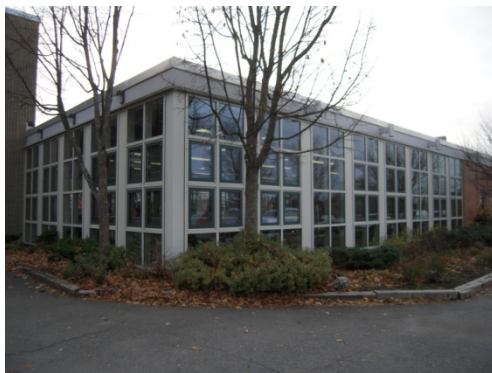
Newer north/east corner of the cafeteria
