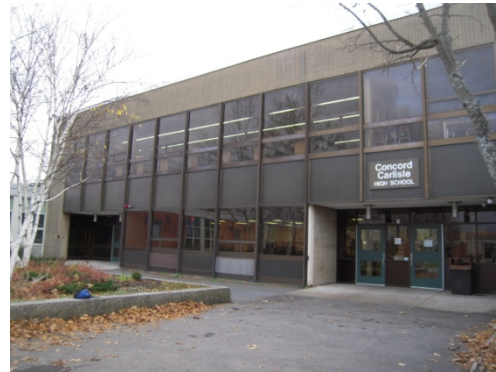
Main entry at two story library building
