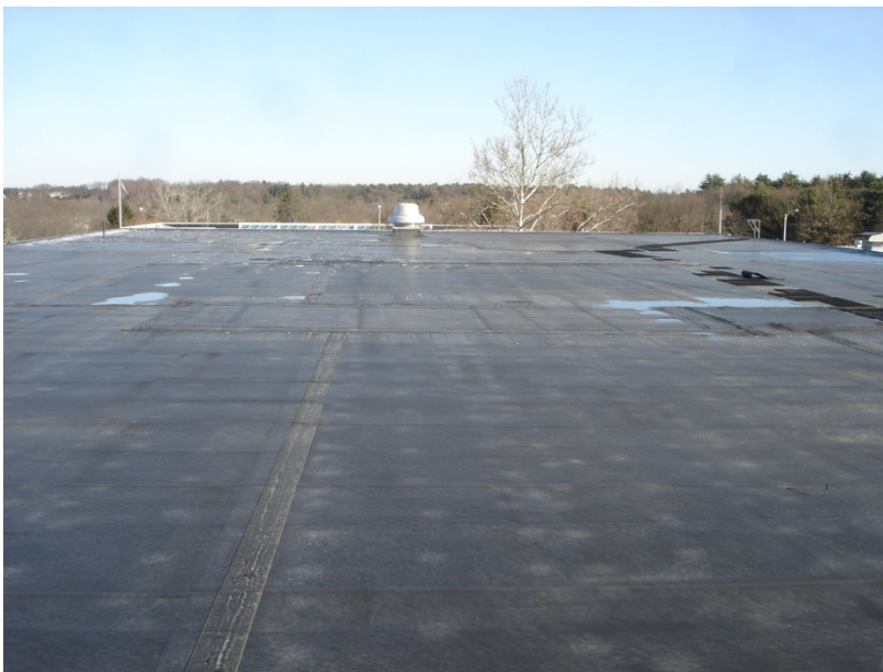
Figure 28. Overall view of EPDM roof.
