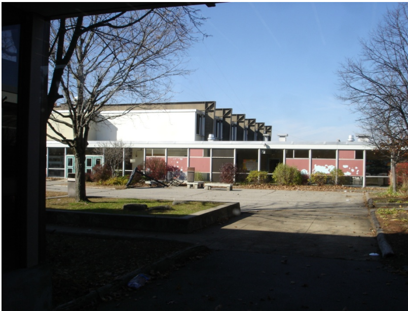
Figure 22. Original curtain wall construction and upper gymnasium structure beyond.
