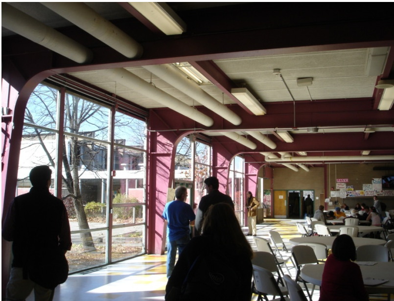
Figure 24. Original curtain wall construction at cafeteria.
