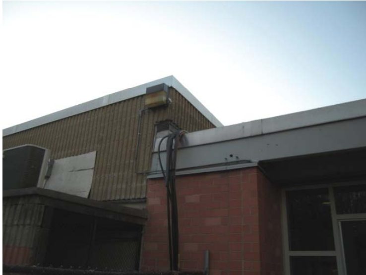
EXPOSED UTILITY LINES
