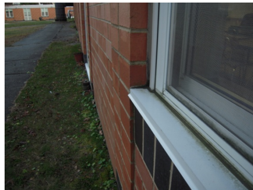
Aluminum sill sloping back towards window
