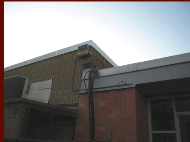
EXPOSED UTILITY LINES
