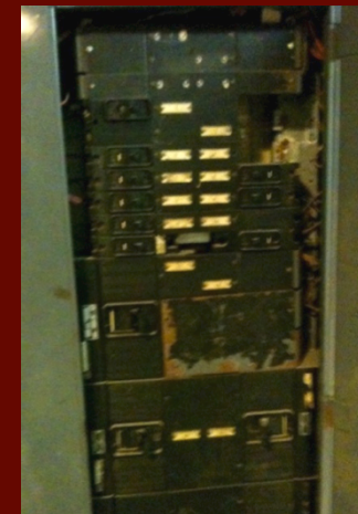
OUTDATED AND DETERIORATING ELECTRICAL PANELS
