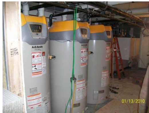
High Efficiency Gas Fired Water Heaters
