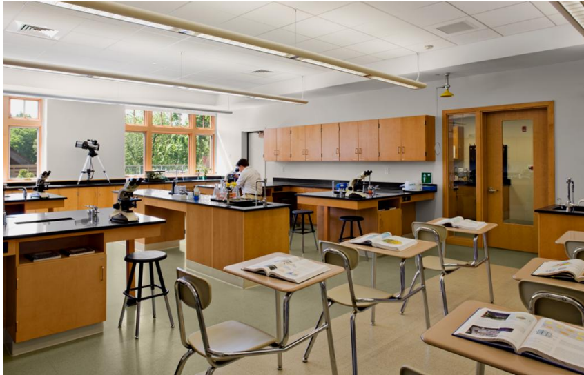
High Efficiency Indirect/ Direct Pendant Lighting
