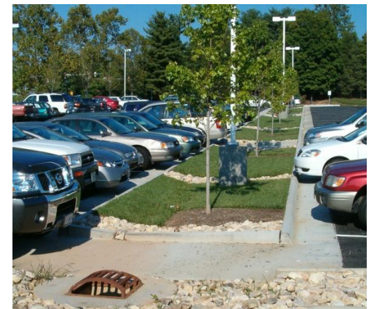
Bio-Retention Stormwater Control
