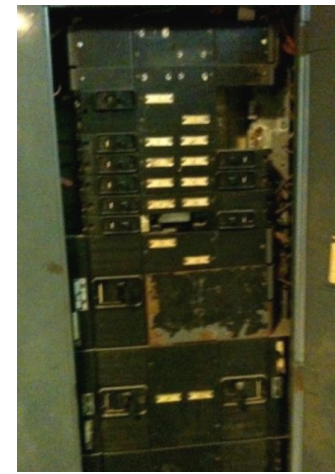
OUTDATED AND DETERIORATING ELECTRICAL PANELS
