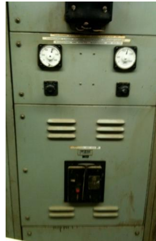
OUTDATED AND DETERIORATING ELECTRICAL PANELS
