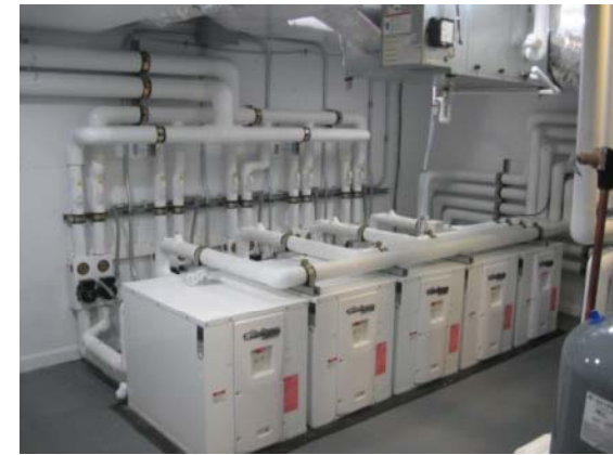
High-Efficiency Chiller
